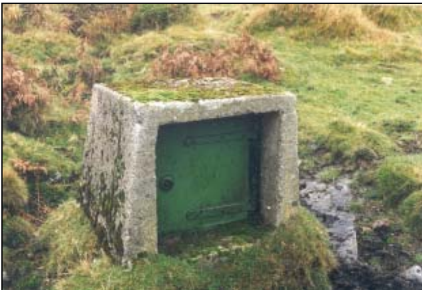
Plate 25: Concrete Telephone Safe with Steel Door
