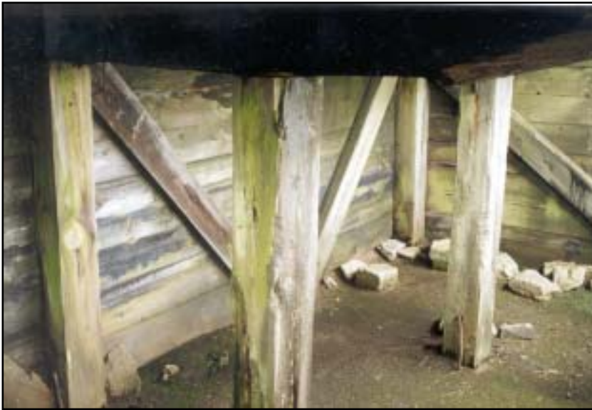
Plate 30: Interior View of Observation Post 3
